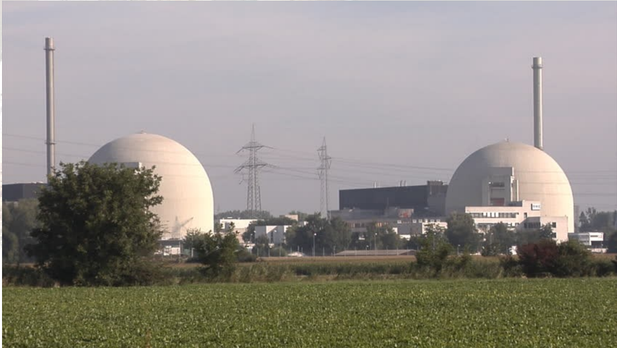
General view of the nuclear power plant in Biblis, near Frankfurt, Germany
