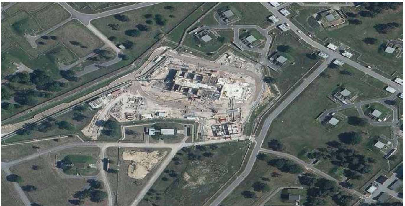
Figure 5: Circinus explosives facility under construction at AWE Aldermaston (Bing).
